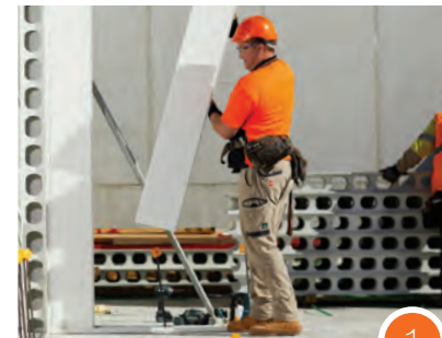
1 Lightweight panels make for easier materials handling
