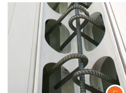
5 Reinforcement placement
