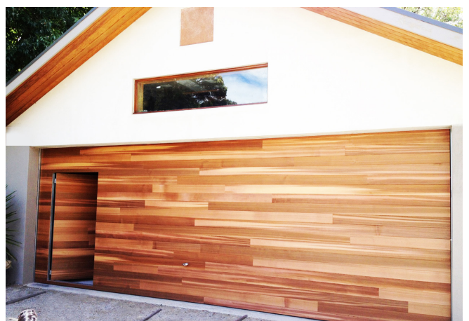
Counterweight Tilt Door with Personal Access Door
